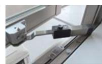
At locations such as rescue entrances, this fitting can be opened at once to 90° with a single action. In an emergency, the cover can be torn from the indoor side, and the window can be easily opened to 90° by turning the knob.
